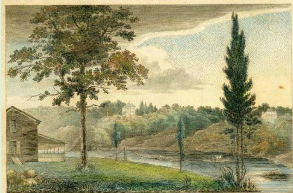
Mendenhall Ferry, Schuylkill, Pennsylvania.
